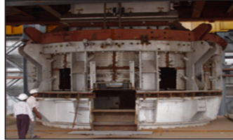
Heavy Equipment Erection
