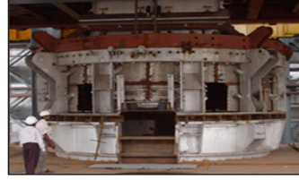
Heavy Equipment Erection
