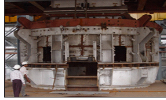
Heavy Equipment Erection
